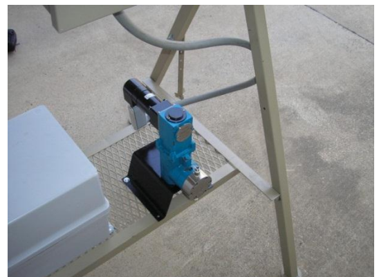
Figure 2.14: Chemical Pump Mounting
